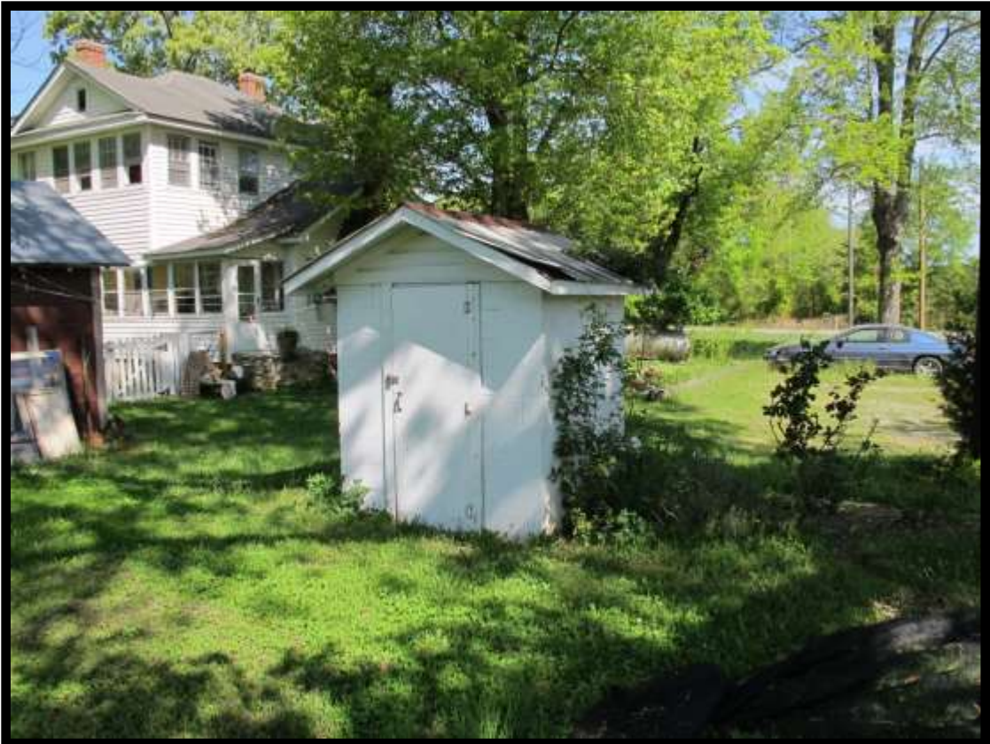
Figure 13: View of Well House Looking Northwest.
