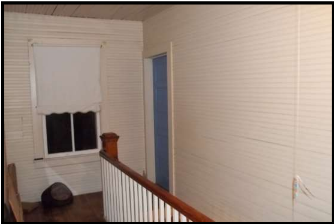
Figure 11: View of the Second Floor Stair Landing.
