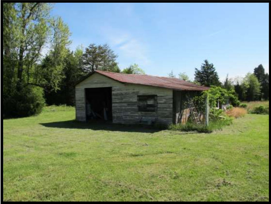
Figure 14: View of Barn Looking Northeast.
