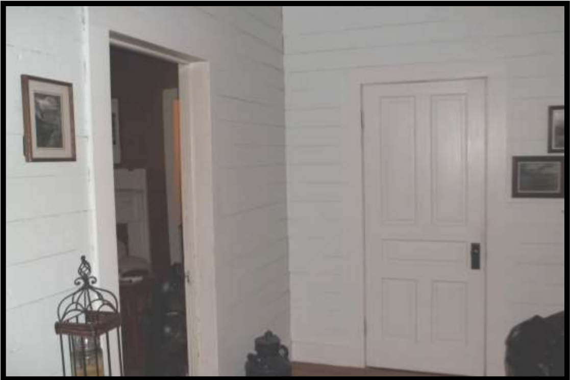
Figure 9: View of an Original Five-Panel Door in the Living Room on the First Floor.
