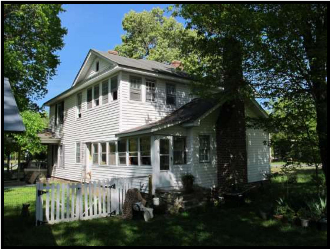
Figure 6: View of the Garrison House Looking Northwest.
